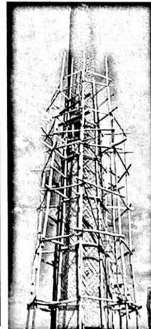
General view of minaret during restoartion
